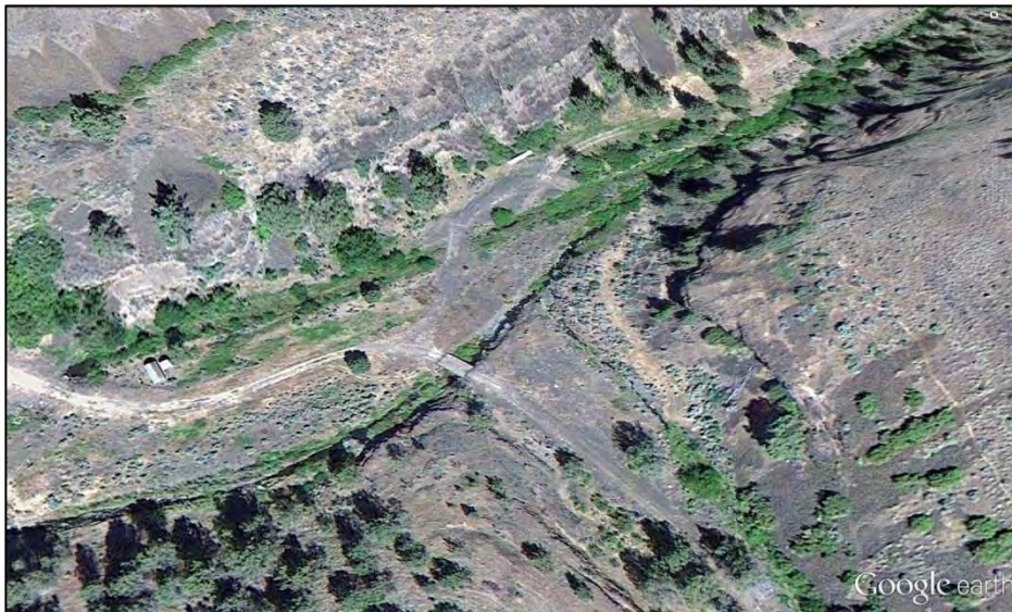
Figure 4-2. Bridge Crossing: Big Pine Hollow Creek
