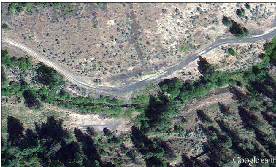
Figure 4-4. Crossing with Adjacent Riparian Road and Evidence of Erosion: Big Pine Hollow Creek
