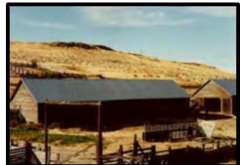
Sheep shearing shed, built before 1918. Carver Ranch photo
